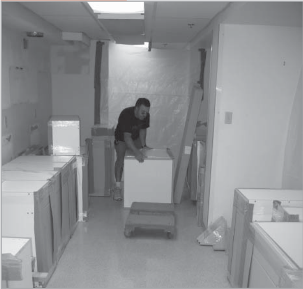
The work has begun.
